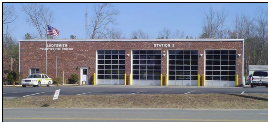
Ladysmith Fire Station
